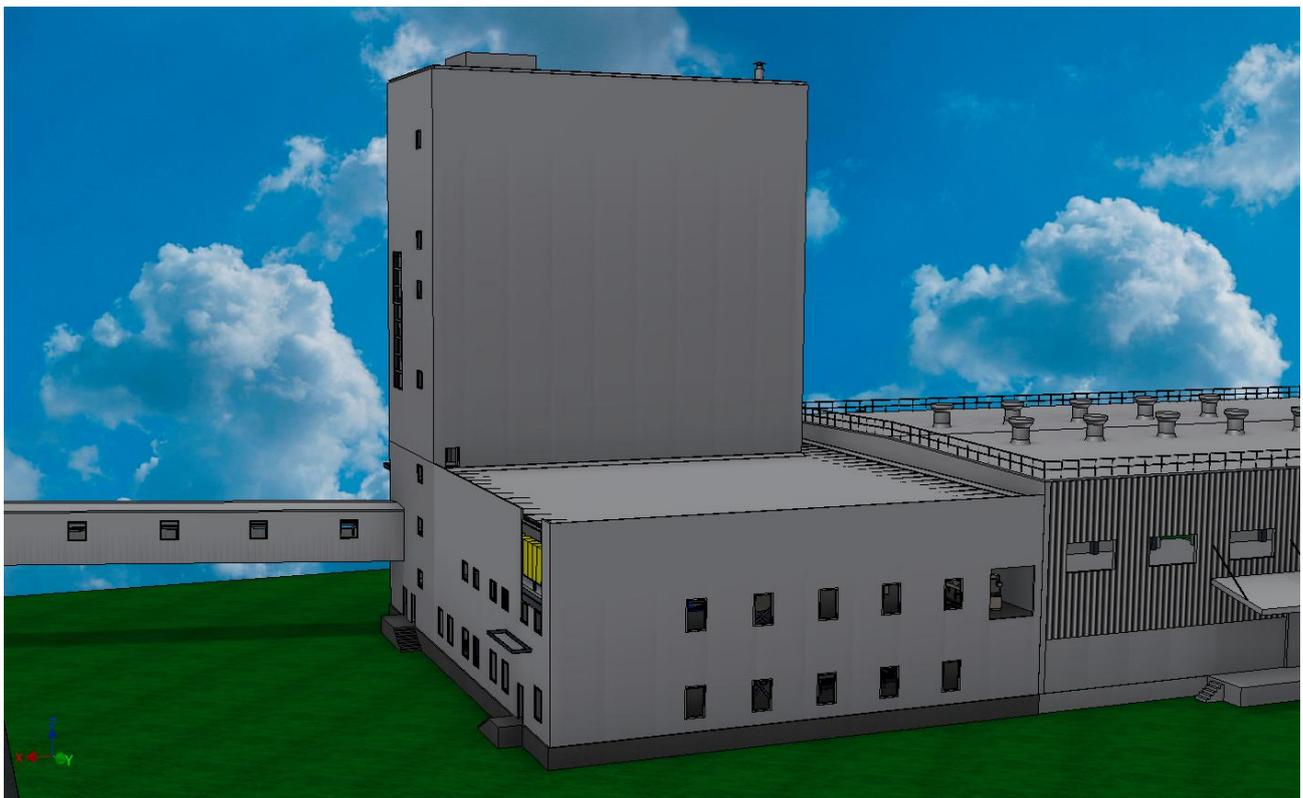
Picture 1: General view of the building object in the planning. Dimensions (WxDxH): 30 m x 36,5 m x 39 m
